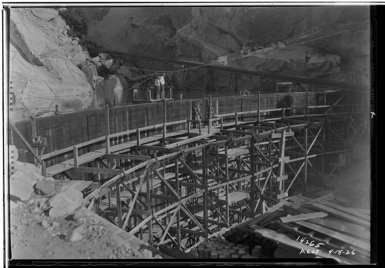
Stevenson Creek Test Dam — view 2
