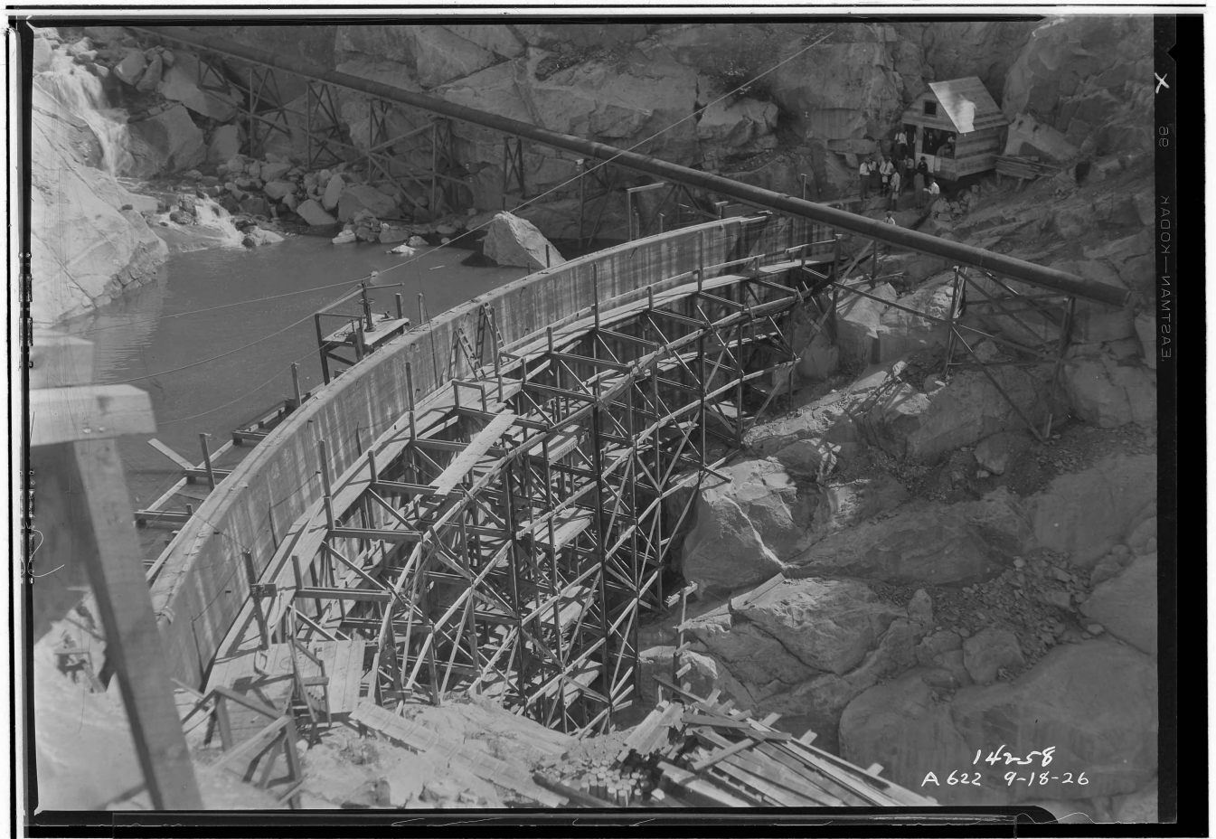
Stevenson Creek Test Dam — view 3
