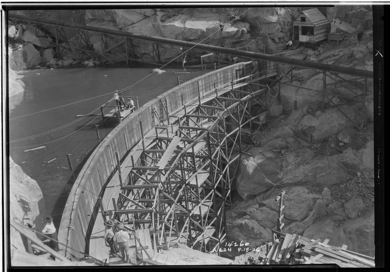
Stevenson Creek Test Dam — view 1
